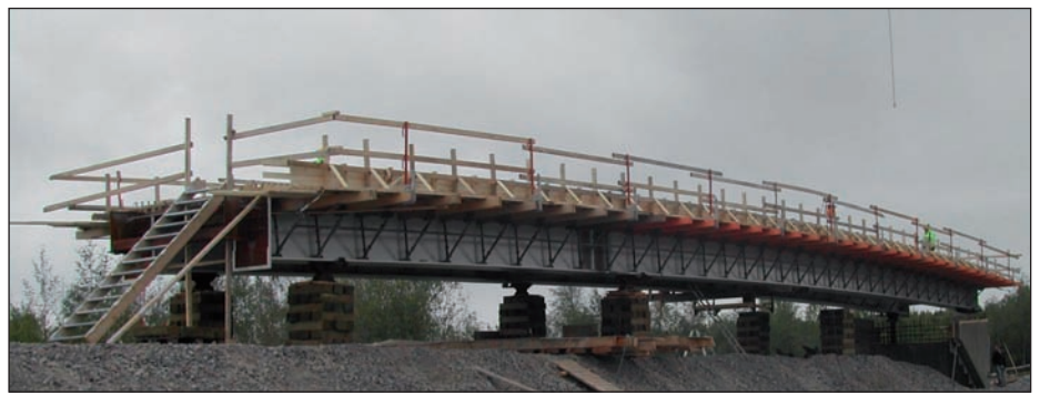
Fig. 6: The bridge superstructure before it was launched in place
